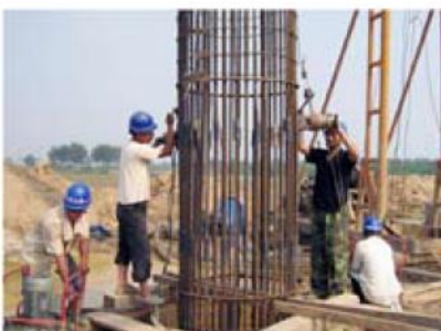
Cold Forged Sleeve for Cage
