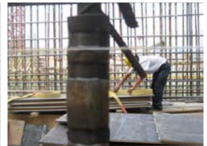
Cold Forged Sleeve Connecting Rebars
