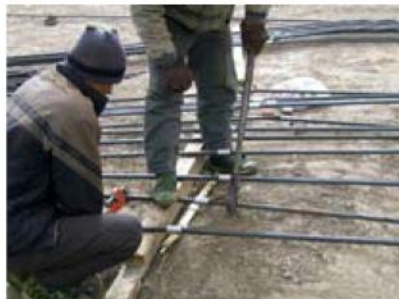
Connecting Rebar Coupler
