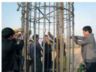
Locking Sleeve Coupler for Cage
