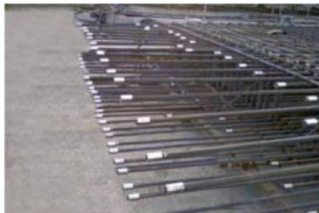
Coupler for Connecting Rebars
