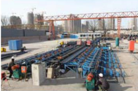
Auto. Rebar Thread End Making Line in site
