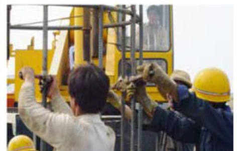
Lifting Rebar Cages
