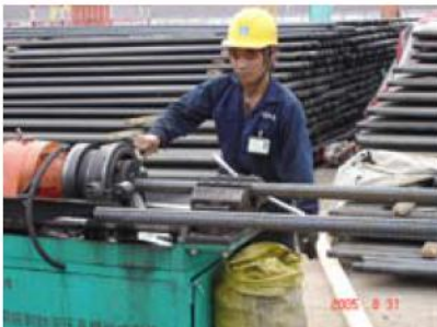
Stripping and Rolling Rebar Thread End
